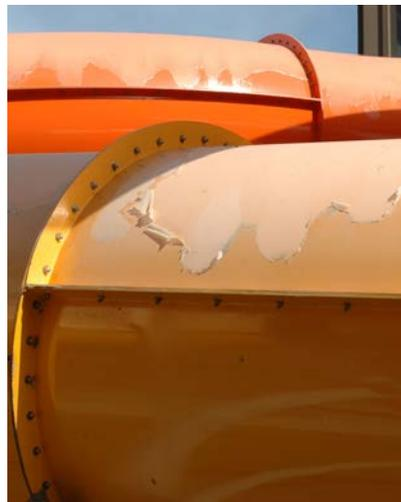
many years, UV exposure can deteriorate the gel coat surface and expose the structural fiberglass layers potentially
